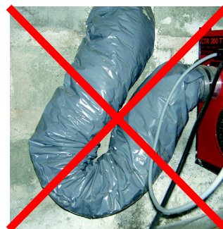
Incorrect installation, sharp bend
