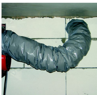
Correct installation, slight bend.
