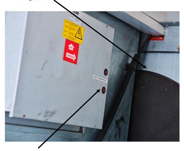
If the machine is overheated it stops and the red lamp (no. 11 on electric cabin) will light up. Let the machine cool, make sure hatches are open, change filters. Open the back doors and reset the red buttons.
